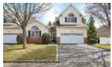
Mount Sinai The Ranches, Updated Amagansett Model w/a full Basement. Gourmet EIK w/ Granite counters. Formal DR & LR w/Fpl, and double sliding doors to private patio. Primary bedroom is on the 1st level w/ 2 wlk in closets and FBth. 2 Car Garag. ML#846630 $769,990
